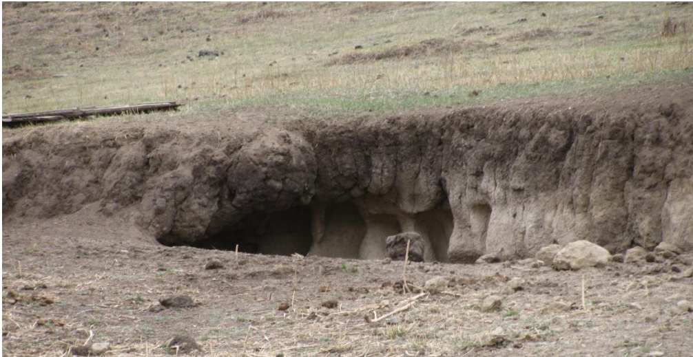
Figure 7 Erosion of upland pasture soils near the Kharaa River. Photo taken 5/11/15
